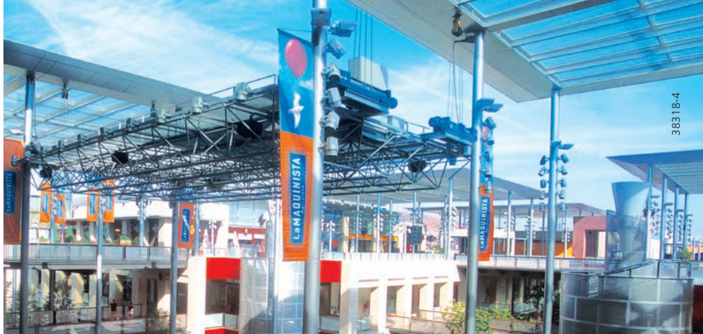
Lifting and lowering a steel and glass roof structure with 4 DH hoist units
